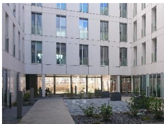
Centre de Services de Nantes - Testing
